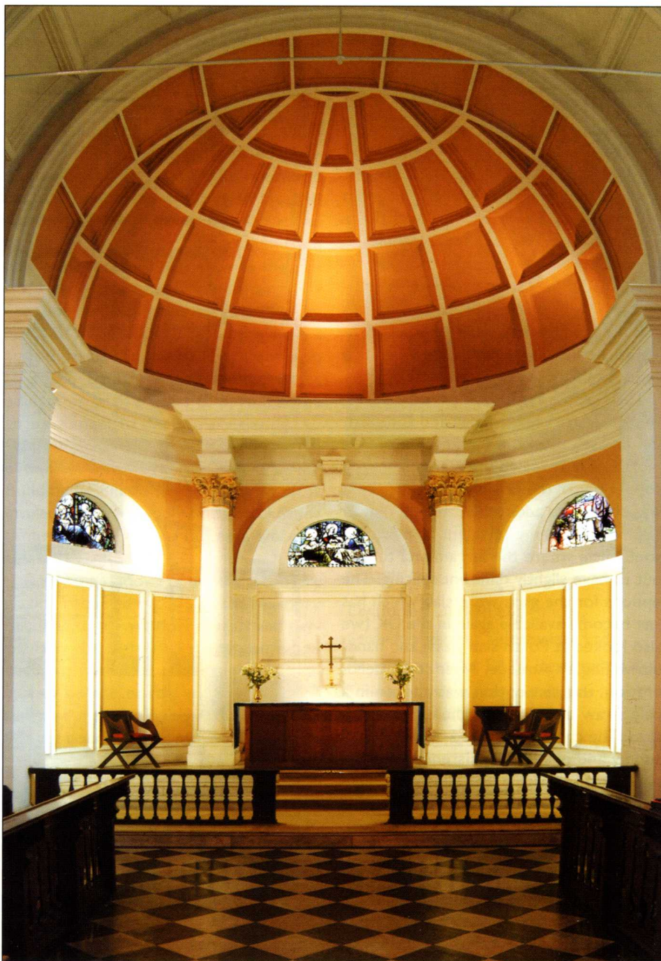
The apsidal east end of the chancel showing the fanlights – can you spot the secondary glazing?
